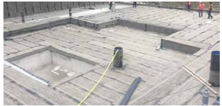
STOPERPROOF H 4,5MM APPLICATION SYSTEM
