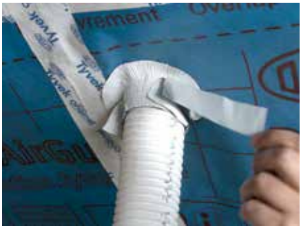
7. Once wrapped around, remove remaining release strip
