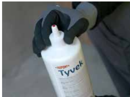
3. Use Tyvek® Primer to stabilise the surface and improve adhesion for the adhesive tape
