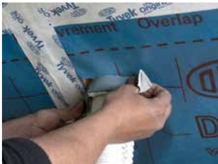
2. Wrap Tyvek® FlexWrap EZ around the pipe base, bonding the exposed adhesive to the pipe
