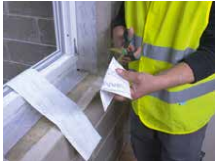
3. Cut half way along the crease
