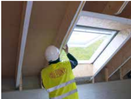
2. Apply tape to all facing surfaces . . .
