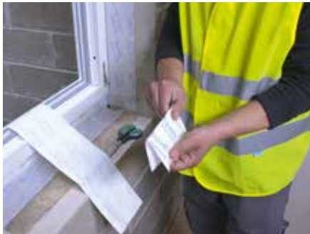
2. Internal corners can be sealed with a separate piece of Tyvek® Plastering Tape. Firstly, cut out a square of tape and fold in half
