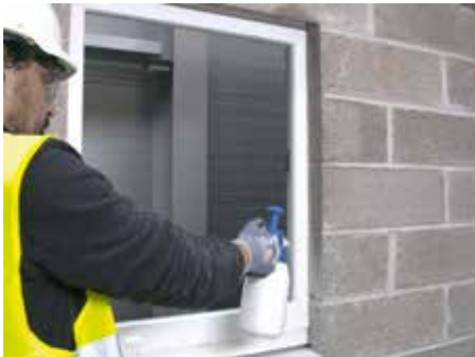
1. Spray water onto external surfaces to effect bond with DuPont™ Insta Stik™
