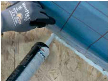
1. Whilst holding the DuPont™ AirGuard® AVCL back, apply a 4-8mm bead of DuPont™ AirGuard® Sealant to the surface
