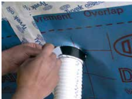
3. Remove the 2nd backing strip
