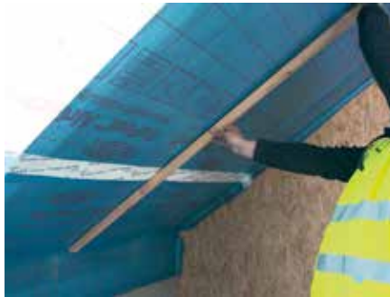
11. Measure battens prior to fixing
