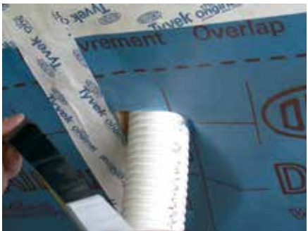
1. Cut a length of Tyvek® FlexWrap EZ, fold in half and remove one release liner strip
