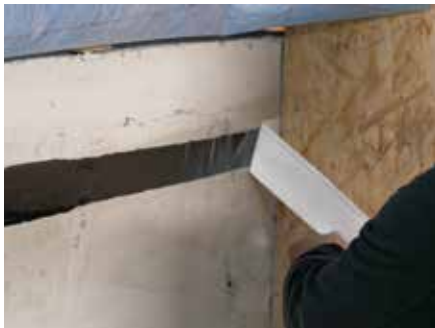
2. Remove backing paper to expose adhesive
