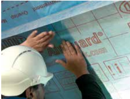
8. AVCL should be pressed firmly against tape
