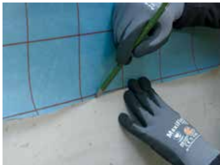
2. Mark out area where primer is to be applied
