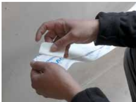
10. Peel away a short length of liner and apply the exposed tape onto the AVCL
