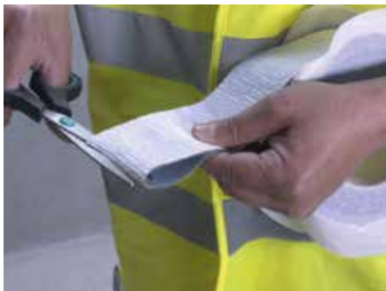
2. Cut off a small length of Tyvek® FlexWrap EZ
