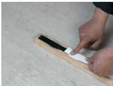
13. Remove release liner
