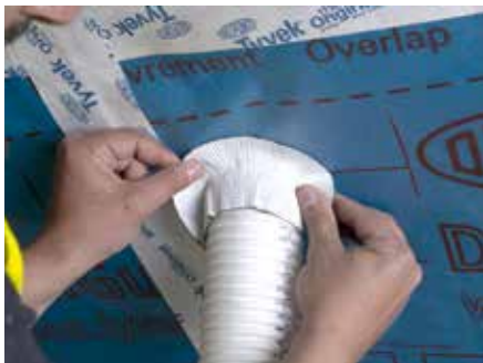
5. Press firmly to establish seal
