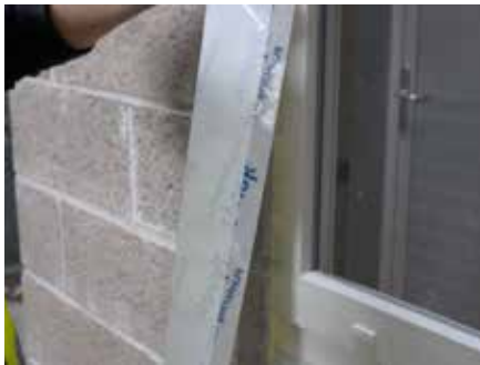
8. Fold a cut length of Tyvek® Window Tape and remove the narrow release strip
