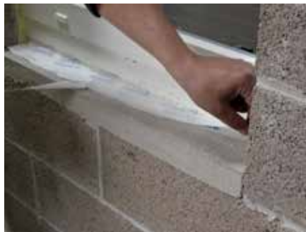
9. Starting at the cill, apply the exposed tape to the frame and remove the remaining backing strip
