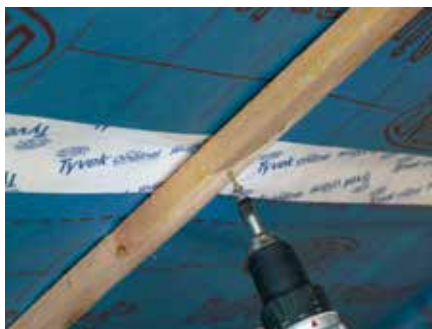
14. Press batten into position and permanently fix
