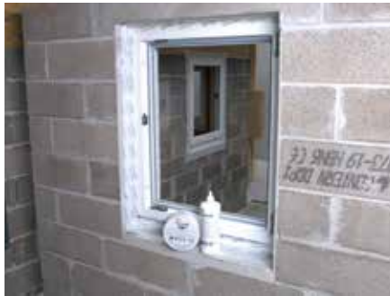
13. Repeat the process for the internal side of the frame and the gap is sealed!
