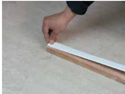
12. Apply Tyvek® Butyl tape to batten
