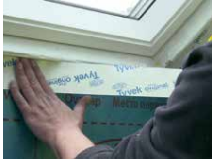
12. Seal tightly around window
