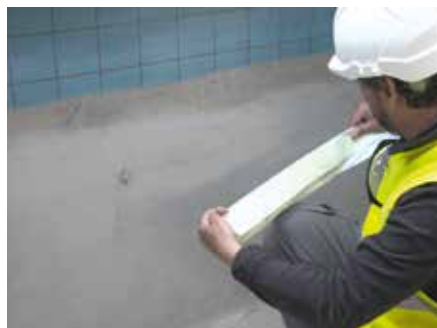
9. Prepare Tyvek® Window/Plastering Tape by folding back along the first split liner
