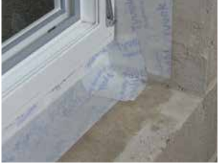
10. Position and firmly press the corner detail into place
