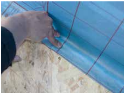
2. Lap the membrane onto the sealant and apply pressure with fingers either side of the bead. Ensure that the sealant is not pressed flat as a bead thickness of at least 1mm should be maintained
