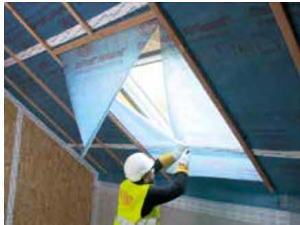
3. Cutting the vertical portion
