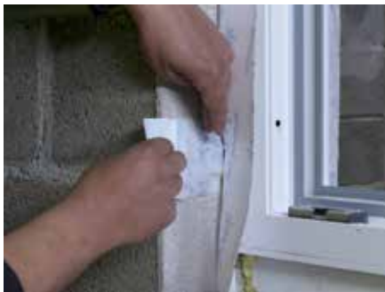
12. Apply Tyvek® Window tape to the window head and reveals taking care to seal and brackets.
