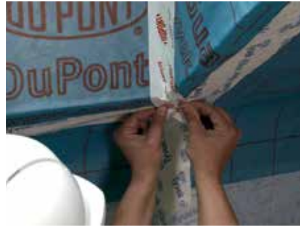
18. . . . a flexible tape that can be used to seal corners and any awkward details
