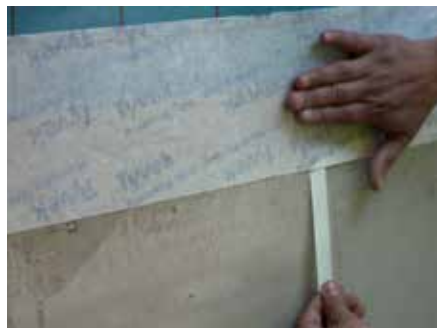
12. Remove remaining release liner and press tape firmly into place
