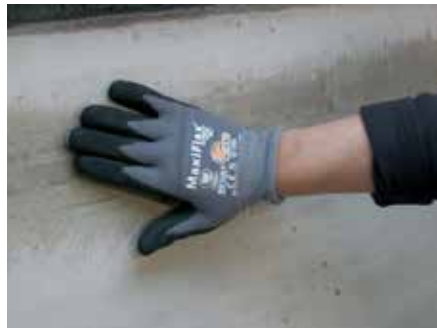
6. After an hour the primer turns transparent
