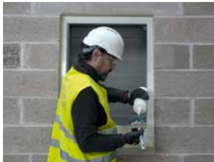
6. Tyvek® Primer can be applied onto the wall surface or directly onto the brush
