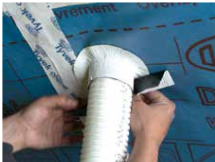
6. Apply a 2nd length of Tyvek® FlexWrap EZ onto the pipe on the opposite side. Try to keep the folded tape flat by 'pinching' together
