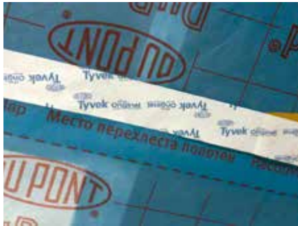
10. Seal laps with Tyvek® Tape (Tyvek® Metallised Tape should be used with DuPont™ AirGuard® Reflective or AirGuard® FR System Tape should be used with DuPont™ AirGuard® A2 FR fire retardant AVCL)
