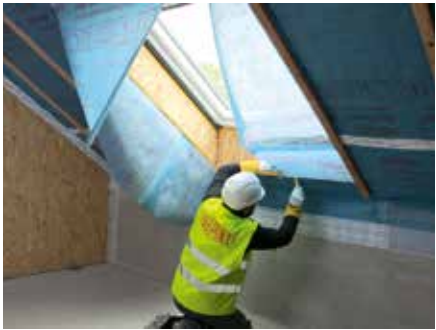
4. Cut AVCL horizontally across foot of window, in line with the reveal edge
