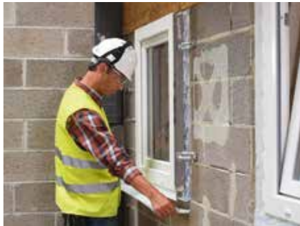
3. Position and secure the window unit and seal the external window/wall junction using Tyvek® Window Tape
