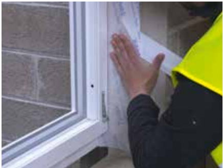
1. The internal window to wall junction can be sealed following the same method described on page 35
