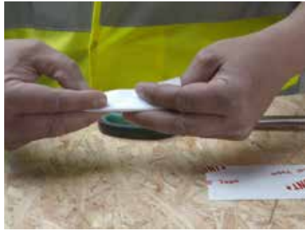
13. Fold DuPont™ AirGuard® Tape in half
