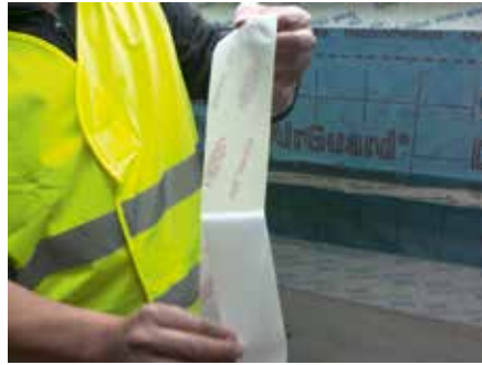
17. Remove release liner from DuPont™ AirGuard® Tape . . .
