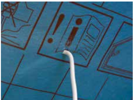
1. Any cables that penetrate a DuPont™ AirGuard® AVCL must be sealed
