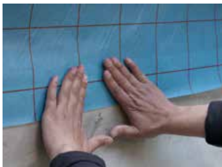
8. Fold DuPont™ AirGuard® AVCL onto primed surface
