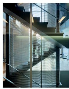
Stairwell cladding using two layers of architectural mesh to create the moiré effect.
