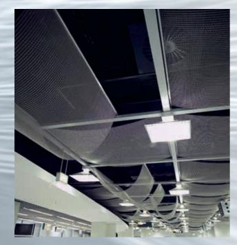
Adjustable mounting system for ceilings with sag.
