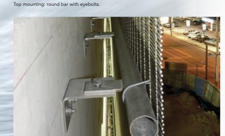
Intermediate mounting: round tube and wire connectors.
