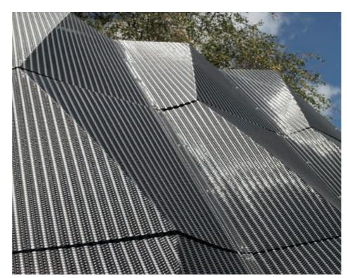
3D mesh façade by Haver & Boecker for mesh cladding with a dynamic effect.
