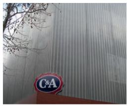
A semi-transparent stainless-steel mesh encloses the existing building and ensures natural lighting. C&A Eco Store, Mainz, Germany.
