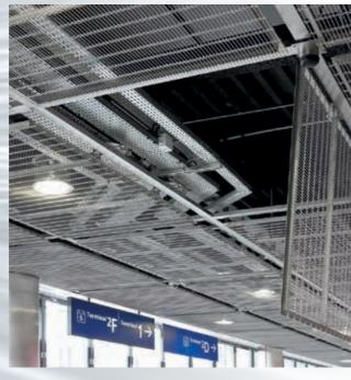
Removable mounting system for ceilings without sag and with framed elements.
