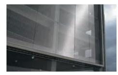
Thanks to its transparency, stainless-steel mesh allows good circulation of air.
