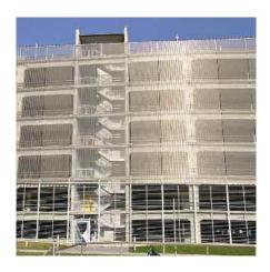
and improving air quality in the space. Architectural mesh can also lessen the cost of a fire protection system.
