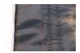
3. Place the hot air nozzle of the machine between the two sheets, and adjust the speed and temperature, depending on ambient temperature
