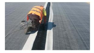
4. Start the automatic welding, adjusting as required to keep the welder on track. Handheld equipment may be helpful to seal difficult areas
