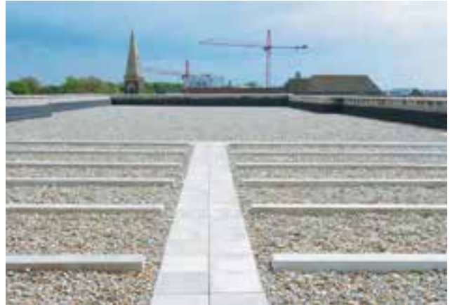
Abb. 24: Bekiestes Umkehrdach
