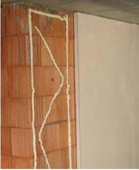
Apply adhesive to wall (or board)
